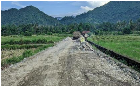
Gambar 2. Proses Penimbunan jalan
